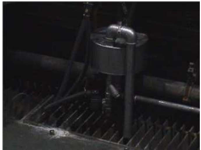
Figure 5. CMC34/10 Conductivity Sensor & the Sensor Holder.
